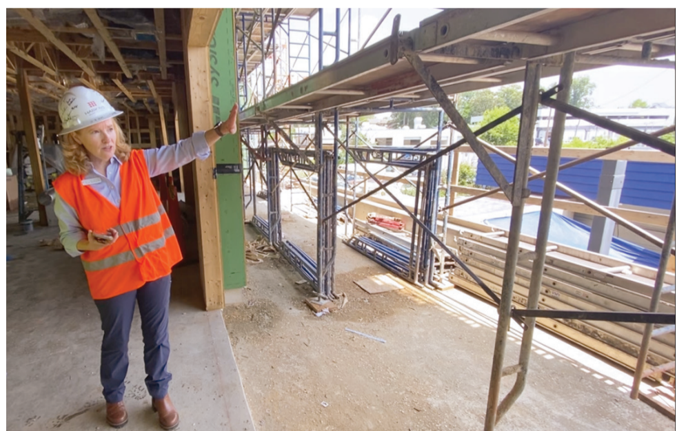
Tara Ruskowski points out where the second-floor balcony will be.
