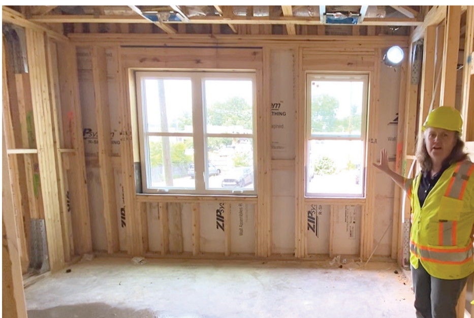
Wendy Baird discussing the windows in this future one-bedroom apartment.
